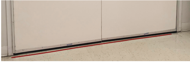
Door Sweep #74918 mounted to a pair of doors.
