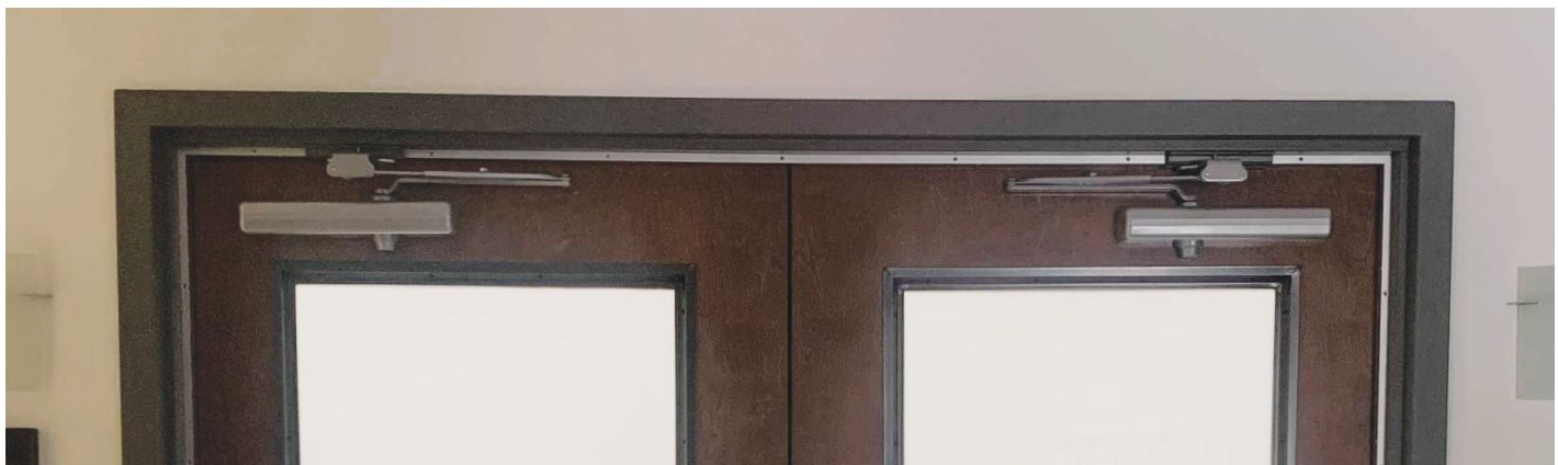
Adjustable gasketing applied to the frame on a pair of conference room doors.
