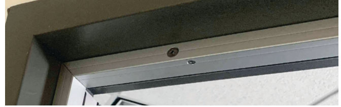
#5077CA Installed on head of frame.
