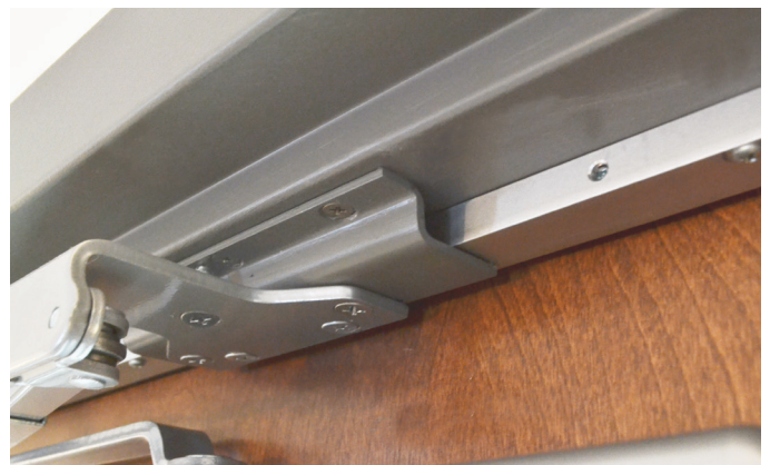
5823SPB installed at the head of the door.
