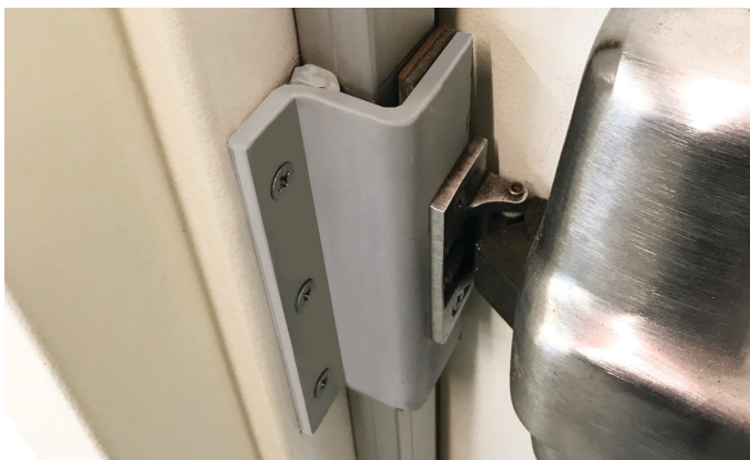
5077SPB installed at the door strike.
