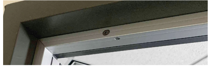
#5077CA Installed on head of frame.
