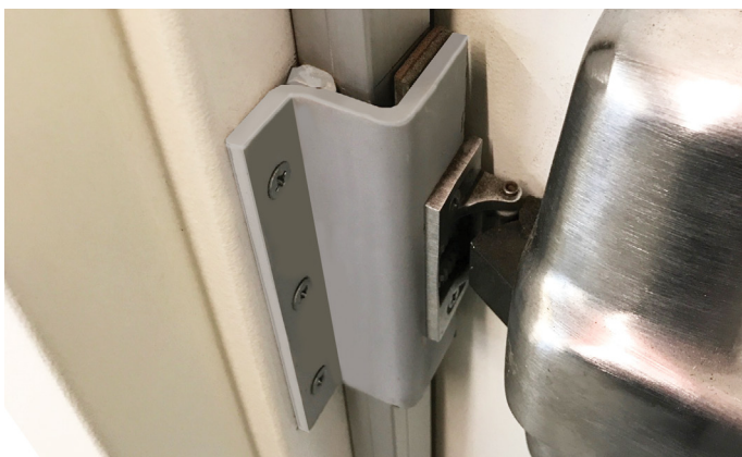
#5078SPB installed at the door strike.
