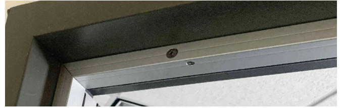
#5077CA Installed on head of frame.
